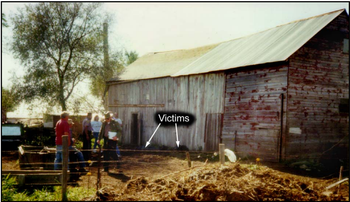
Photo 1 -- View of pen area and adjacent barn showing lack of barriers or protective structures.
